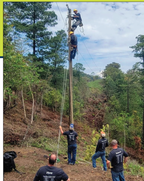
LEFT: From the National Rural Electric Cooperative Association archives, farmers in the 1930s set a pole by hand with pulleys. RIGHT: The Minnesota-Iowa linemen had to employ old-fashioned methods in Guatemala without the convenience of a bucket truck. (NRECA archives/Joe Miller)
