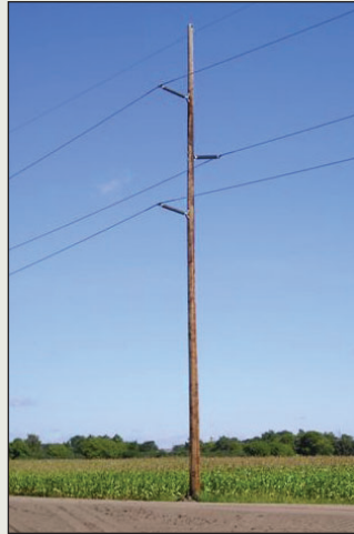
69-kV/115-kV transmission structure
